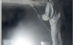
Shotcrete: 100% quality. Only 25% downtime.
